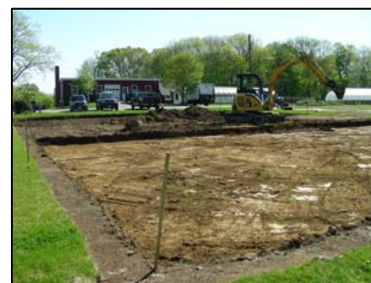
Figure 1. Excavation of soil to a depth of 12".
