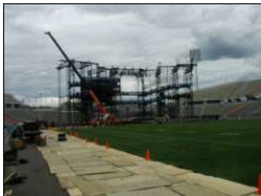
Fig. 1. Portable roadway systems can cause significant turfgrass damage when used for extended cover periods.
