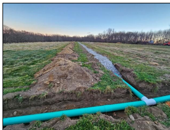
Indoor organic strawberry production being set up (Left). Tile drainage being installed at the UConn Orchard site (Right). Photos by Evan Lentz.
